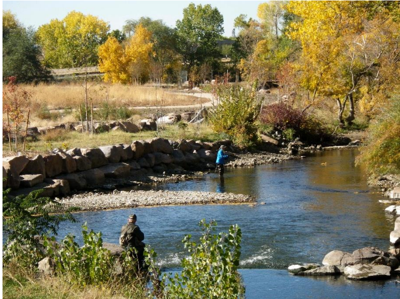
Constructed rock structures in the Ogden River helped improve fish habitat and attracted fishers. River Restoration
